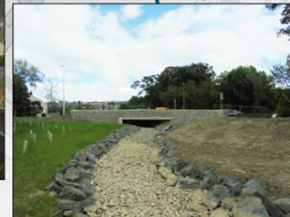
New reinforced concrete bridge and improved A707/A708 junction
