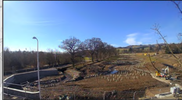
Re-meandered burn and new Angles Field park during landscaping works
