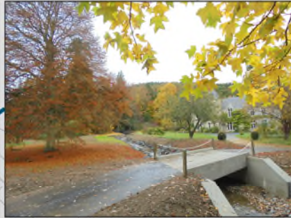
Burn restoration and new reinforced concrete bridge
