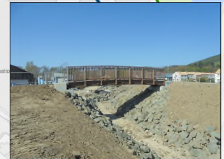
3 new Ekki timber footbridges raised above the 1 in 200 years flood level. Can remain open during high flow events
