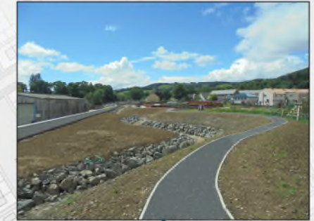
Flood wall, flood embankment and re-meandered burn next to Bannerfield playpark
