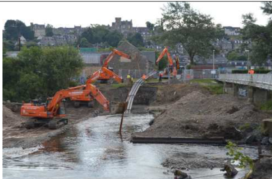
Above: River crossing works, July 2014. Courtesy of J. McCallum
