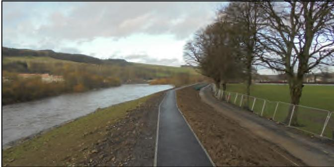
**Work Section 12:** A flood embankment has been constructed and erosion protection works undertaken on the river bank. A new high level footpath has been constructed on top of the embankment which has excellent views to the river. The existing track / footpath remains at a lower level beside the trees.
