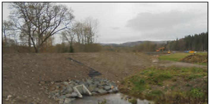
**Work Section 2:** An embankment has been constructed at the western end of Old Mill Farm. This will tie into the A708 flood defence wall, protecting this low lying area from flooding from the Ettrick and Yarrow Waters. The culvert in the foreground acts as a flow control from the Ettrick Water into the Mill Lade.
