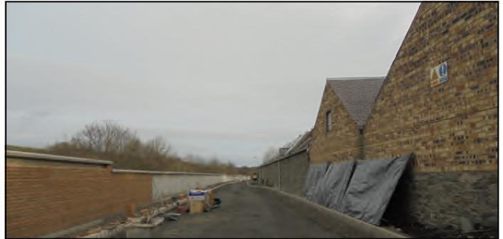
**Work Section 14:** A flood protection wall has been constructed along Riverside Road. This wall will be faced with brick to echo the mill buildings - the brick will continue along the length of wall visible in this photo. There is a footpath on the river side of the wall. This wall protects Riverside from a 1 in 500 years flood.
