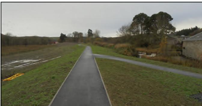
**Work Section 3:** An embankment has been constructed running parallel to the Philiphough Mill Lade, turning towards high ground (i.e. Works Section 2) just before the Murray's Cauld. Defences have been constructed all the way to the main town bridge. The footpath network has also been upgraded.
