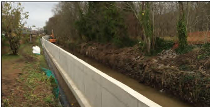
**Work Section 6:** A flood protection wall has been constructed along the Mill Lade to protect properties in this area from flooding from the Ettrick. This wall also has the effect of narrowing the Mill Lade which will increase the velocity of flow which should improve the environmental condition of the lade.
