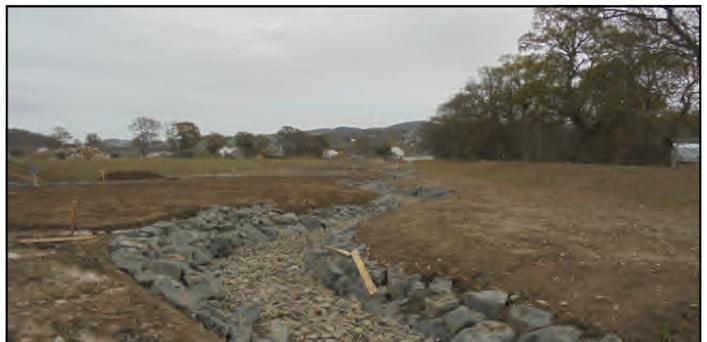
**Work Section 28:** A new meandering channel for the Long Philip Burn has been created through the Angles Field and contained between two new embankments. This forms a new area of parkland: a path will run through the park connecting to Bridge Street footbridge to the east & the Three Brethren to the west.
