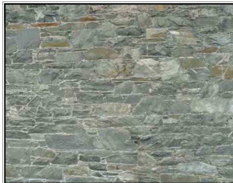
Random rubble masonry (local Selkirk stone)
