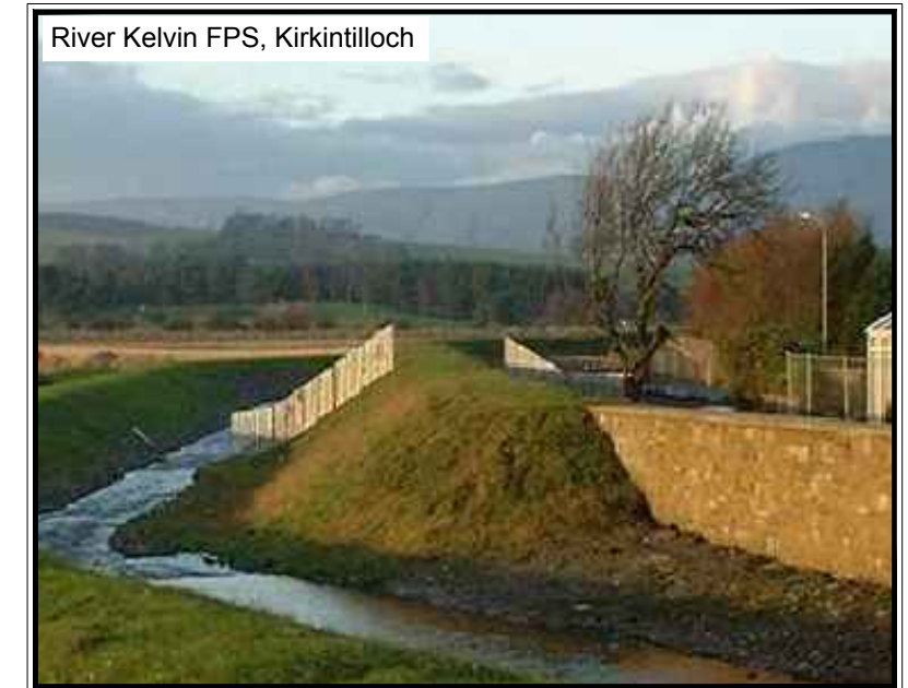
Typical floodwall / embankment transition
