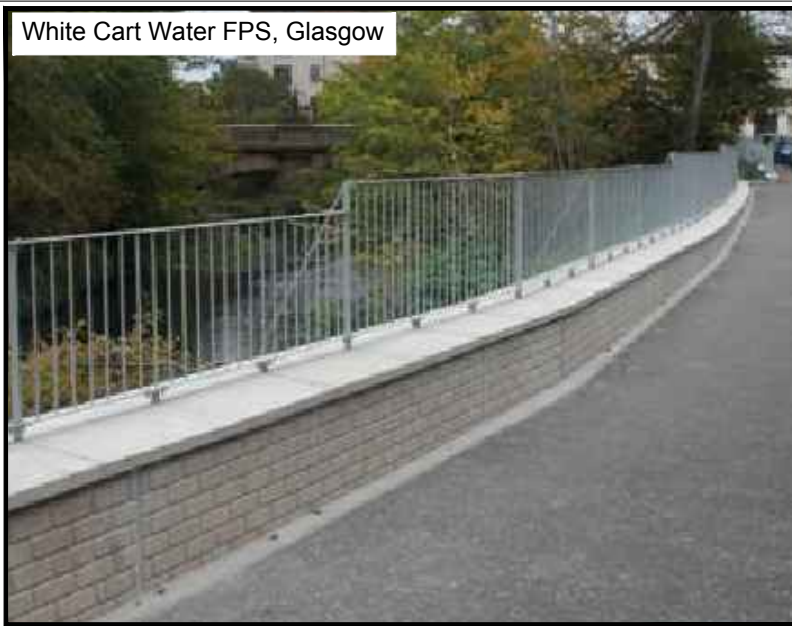
Brick formed concrete finish
