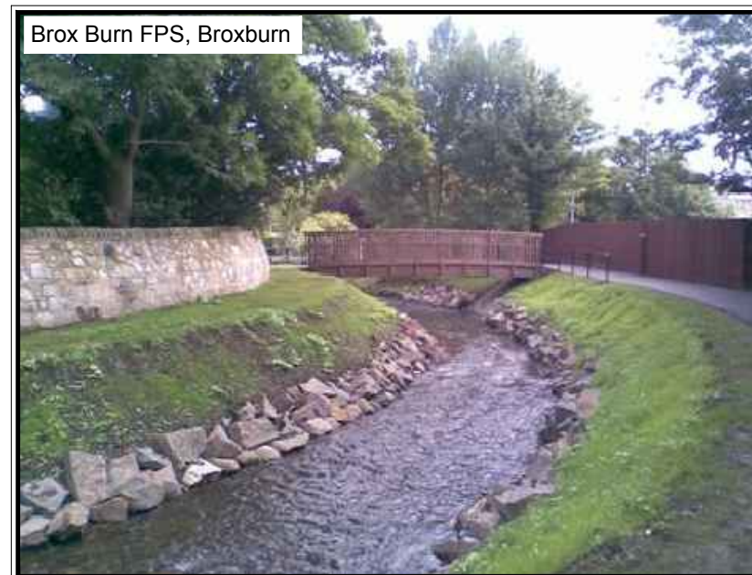
Timber footbridge & erosion protection using rip-rap and geotextiles
